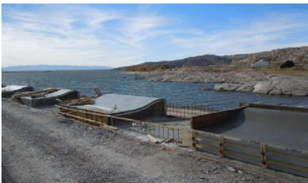
Pathfinder Modification Project ogee weir construction, 2011
